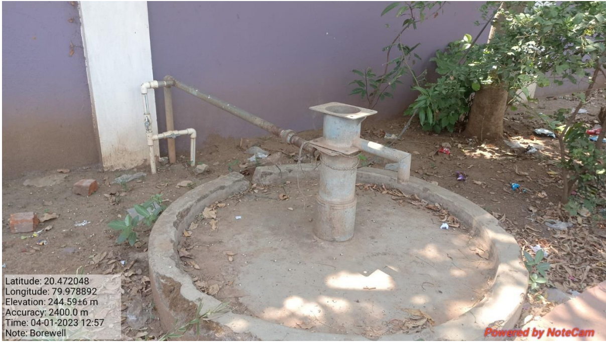
Rain water flow from campus ground increases water level of Borewell
